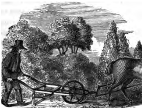
[Fig. 20. Implement in use at Blithewood for cleaning gravel roads.]
